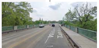
VIEW FROM ROADWAY FACING NORTH
