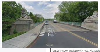
VIEW FROM ROADWAY FACING SOUTH
