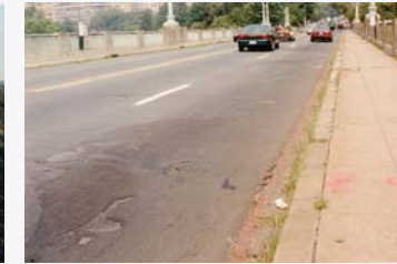
Bridge before 1995 rehabilitation - DDOT Historic Collections
